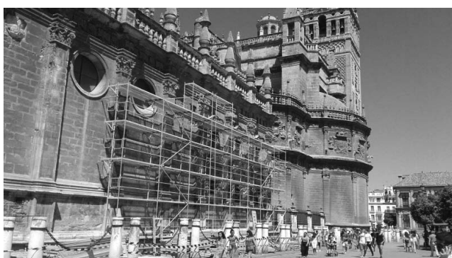
Installation of scaffolding. Phase 1ª. Square of Triumph
