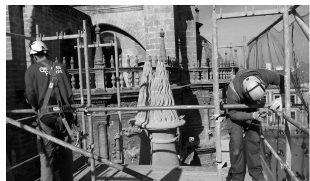
Installing scaffolding on deck
