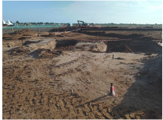
Figure 10. Excavated pits of 0.9m deep
