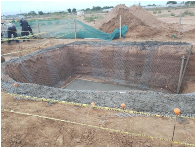
Figure 13. Soil nailing used with chain link for 1.6m pit
