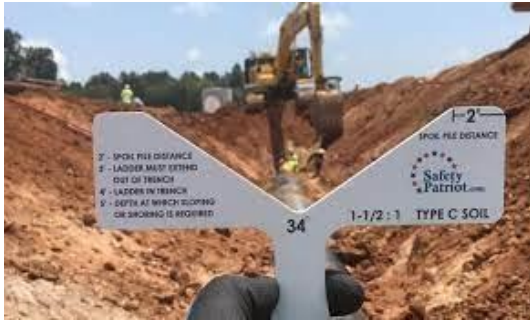
Figure 1. Sloping of excavation edges
