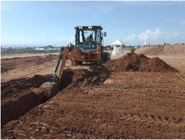
Figure 9. Backhoe excavating a trench 0.9m deep.
