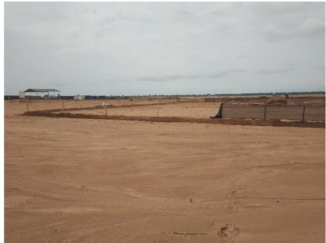
Figure 14. Barrier mesh installed to restrict access
