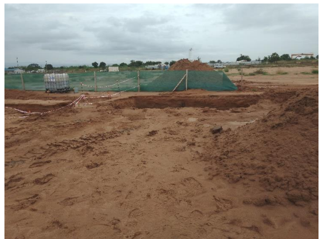
Figure 12. Excavated pit 1.6m deep for septic tank
