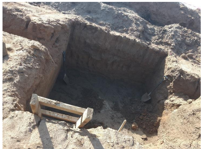
Figure 16. Wooden ladder used for access
