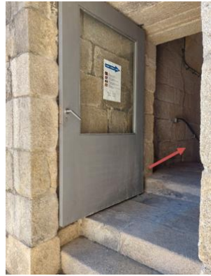
Figure 4. Access to the North Tower
