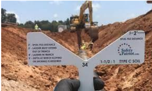
Figure 1. Sloping of excavation edges
