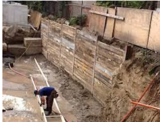
Figure 4. Shoring of lumber installed
