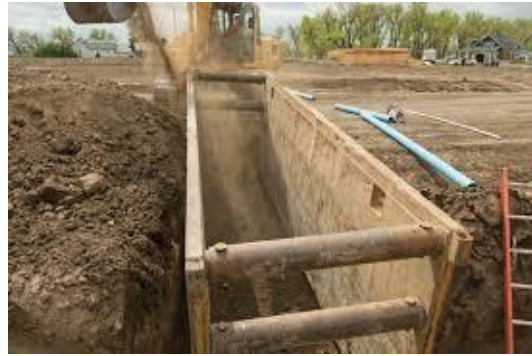
Figure 2. Use of trench box
