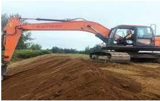
Figure 1. Sloping of excavation edges
