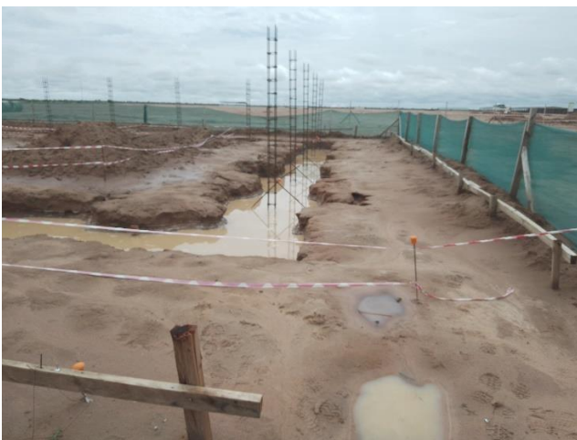
Figure 11. Trench 1.2m deep submerged with water
