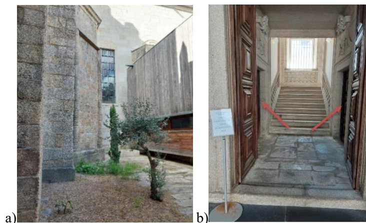
Figure 3. a) The confrontation between the stone facade and the wooden façade; b) Wooden doors accessing the Nasoni staircase
