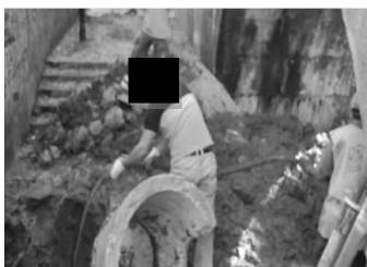
Figure 2 - Attaching the hose cleaning the collector.
