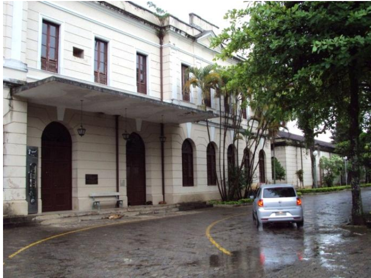
Figure 3 – Main access to Station of the Leopoldina Railway
