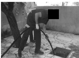
Figure 1 - Cleaning with support from a car
