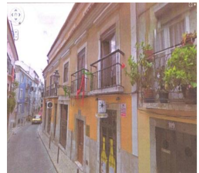
Figure 1 – Building in Rua da Rosa, Lisbon
