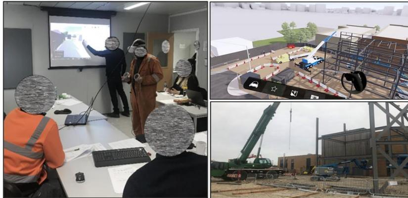
Figure 6 VR Planning - Crane Locations & On-site Crane Arrangements
