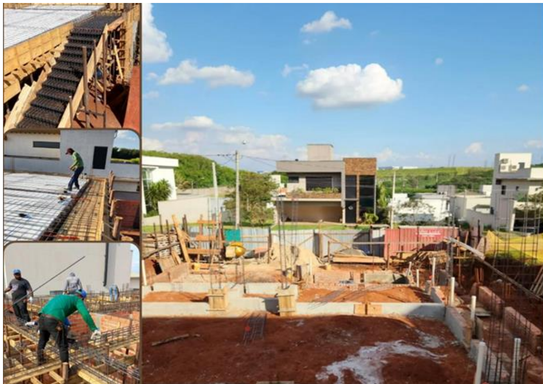
Figure 1: General view of the construction site during various stages of the execution of the foundations and reinforced concrete structures
