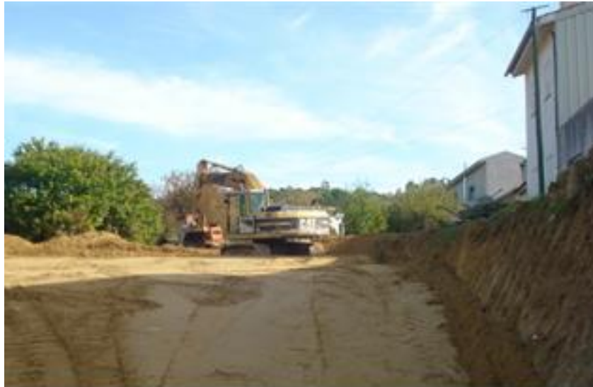
Figure 4. Swivel and cylinder used on site (Henrique, 2017).
