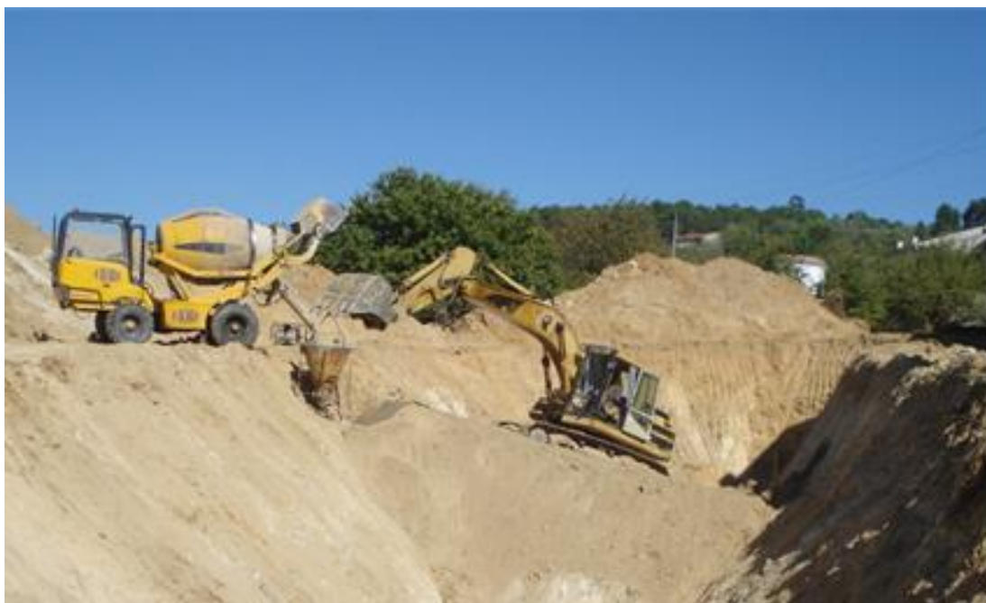
Figure 6. Certified equipment used on site (Henrique, 2017).
